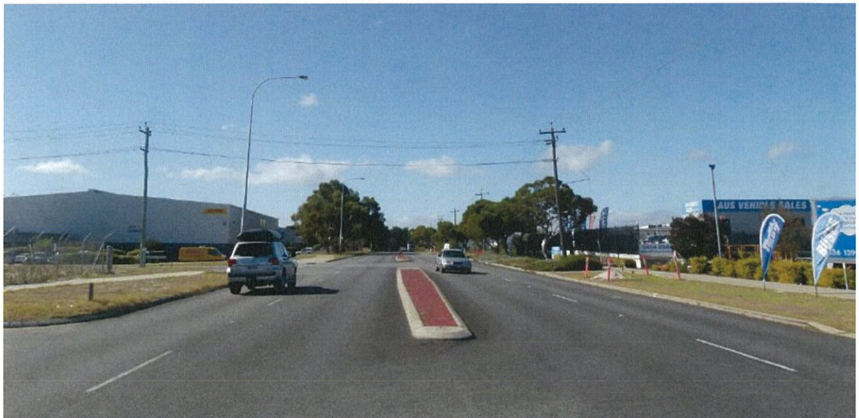
Photograph 3 – The dual-lane carriageway of Collier Road.
