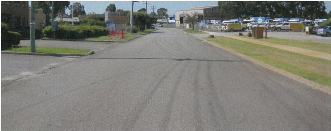
Figure 17: Fairford Street adjacent to the development site - looking north
