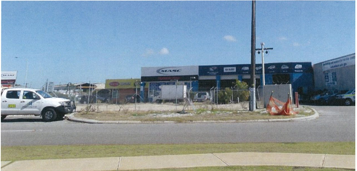
Photograph 2 – The subject site viewed from Fairford Street
